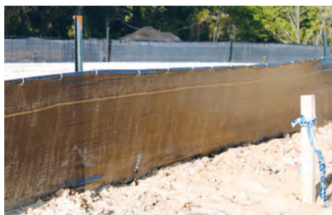
Construction sites use geotextiles to help control erosion and drainage.
