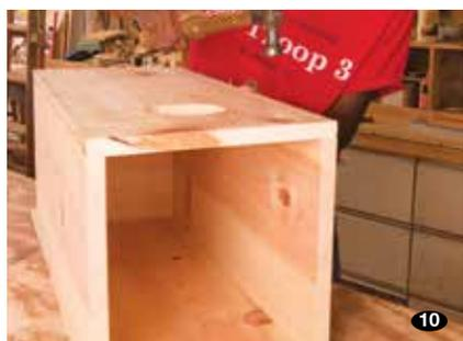
10. Attach the front (with the hardware cloth on the inside) by nailing through the front into the sides and floor.
