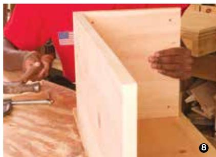
8. Attach the floor to the right side and the back panel. Nail through the side and through the back into the floor.
